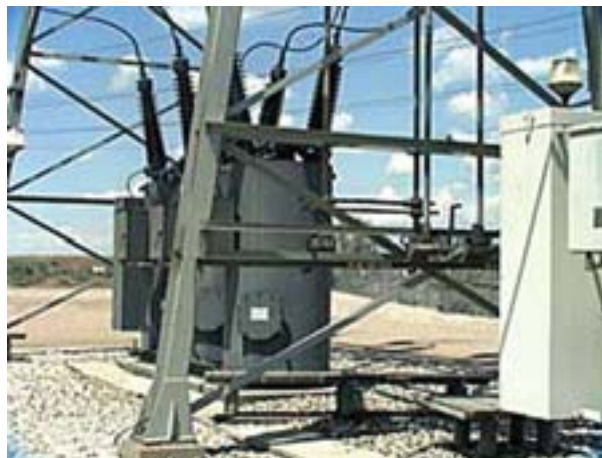
Oil circuit breaker
