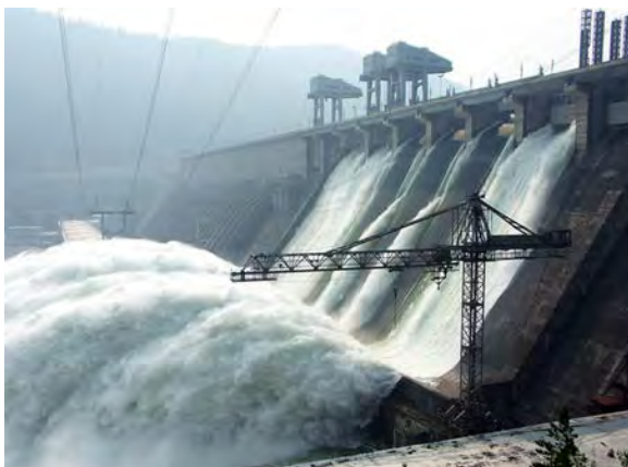
Figure 7.38 Hydroelectric facility (credit: Denis Belevich, Wikimedia Commons)
