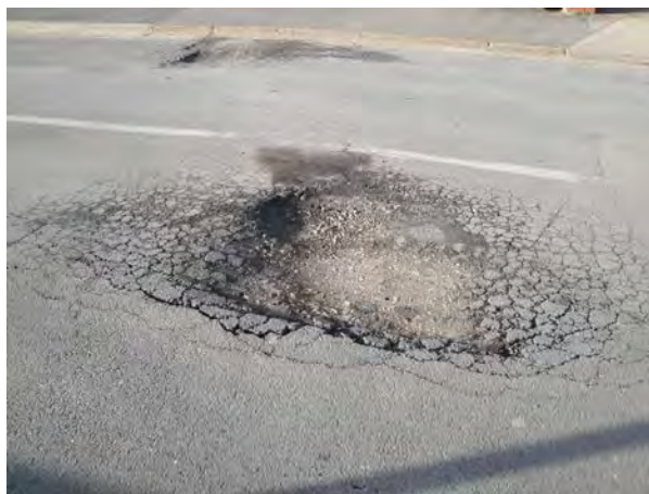
Figure 13.14 Thermal stress contributes to the formation of potholes. (credit: Editor5807, Wikimedia Commons)
