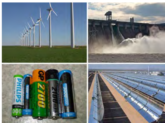
Figure 21.8 A variety of voltage sources (clockwise from top left): the Brazos Wind Farm in Fluvanna, Texas (credit: Leaflet, Wikimedia Commons); the Krasnoyarsk Dam in Russia (credit: Alex Polezhaev); a solar farm (credit: U.S. Department of Energy); and a group of nickel metal hydride batteries (credit: Tiaa Monto). The voltage output of each depends on its construction and load, and equals emf only if there is no load.
