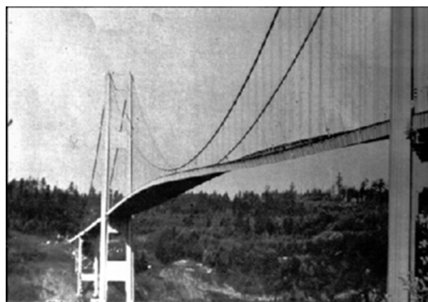
Figure 16.28 In 1940, the Tacoma Narrows Bridge in Washington state collapsed. Heavy cross winds drove the bridge into oscillations at its resonant frequency. Damping decreased when support cables broke loose and started to slip over the towers, allowing increasingly greater amplitudes until the structure failed (credit: PRI's Studio 360 , via Flickr)
