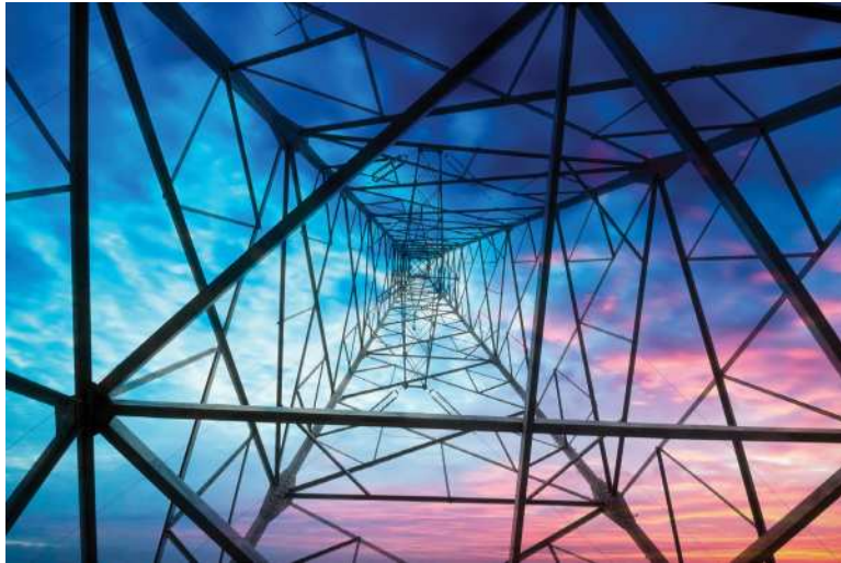
FIGURE 11-1 Trusses are rigid networks of simple two-force members and provide the framework for many structures such as this tall tower. Each member of this tower is long relative to its cross section, so any that is loaded in compression is susceptible to buckling. Care must be taken to ensure that no single member of this structure buckles resulting in a sudden and catastrophic failure of the entire structure.
