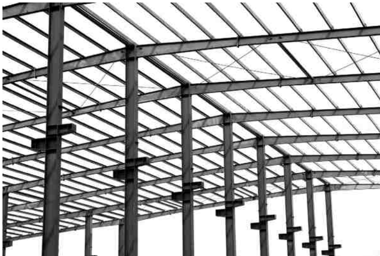
FIGURE 7–1 (See color insert.) Elements loaded in bending require more analysis than those with simple axial loads, and proper calculation and design is critical. Look at all the beams in this building, and consider the serious responsibility of the designer to assure that, once completed, these beams can safely support the roof panels, the roofing material, and all other loading.
