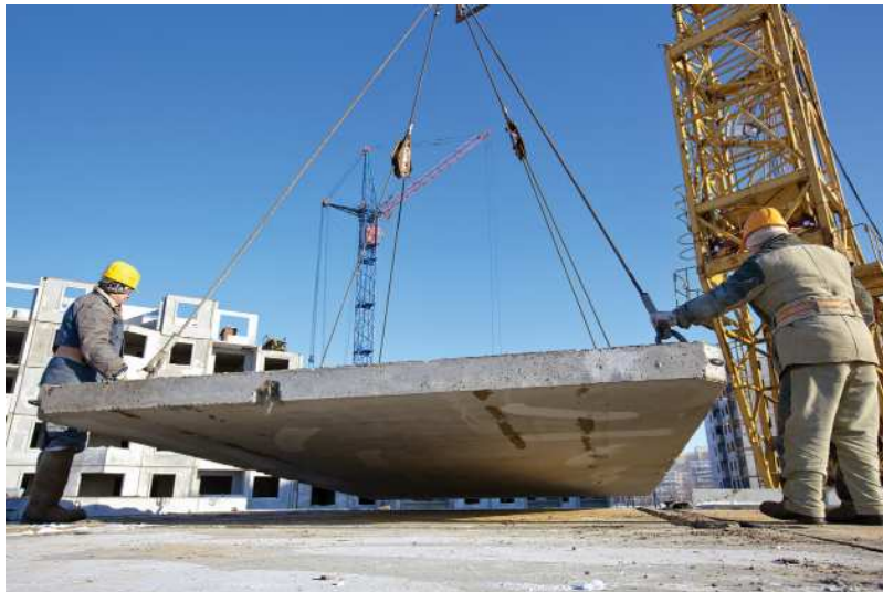
FIGURE 1-1 The concepts of strength of materials are critical in many applications, including this one where workers assure that this concrete element is ready to be lifted into place where it will serve as a critical piece of a multistory structure.
