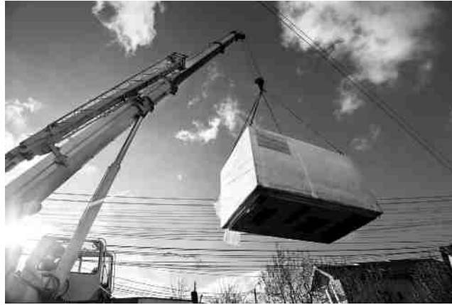
FIGURE 10-2 Crane boom loaded in bending and compression.
