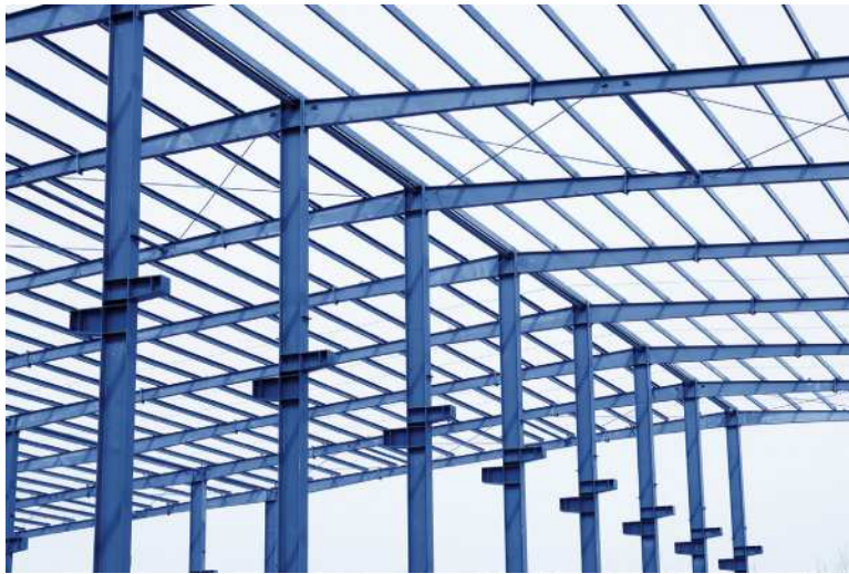
FIGURE 7-1 Elements loaded in bending require more analysis than those with simple axial loads, and proper calculation and design is critical. Look at all the beams in this building, and consider the serious responsibility of the designer to assure that, once completed, these beams can safely support the roof panels, the roofing material, and all other loading.
