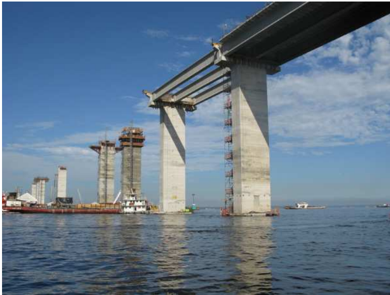
FIGURE 5-1 A bridge under construction shows vertical supports in place where beam reactions will occur. One can see that the effect on each beam in the completed bridge will vary with respect to position relative to those supports. In this chapter, we will learn to quantify what is happening internally along the length of a loaded beam so that, in a subsequent chapter, we will be able to calculate stress and deflection in beams.
